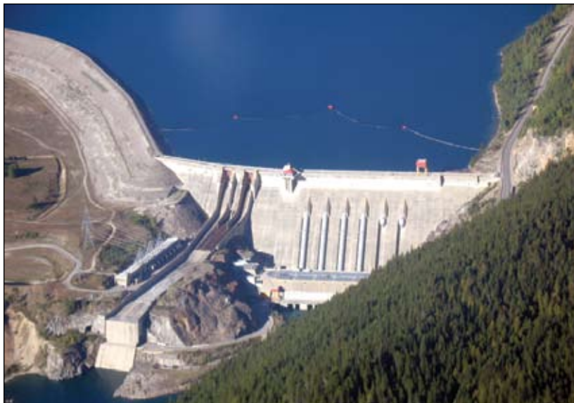
Revelstoke Hydro Dam.
