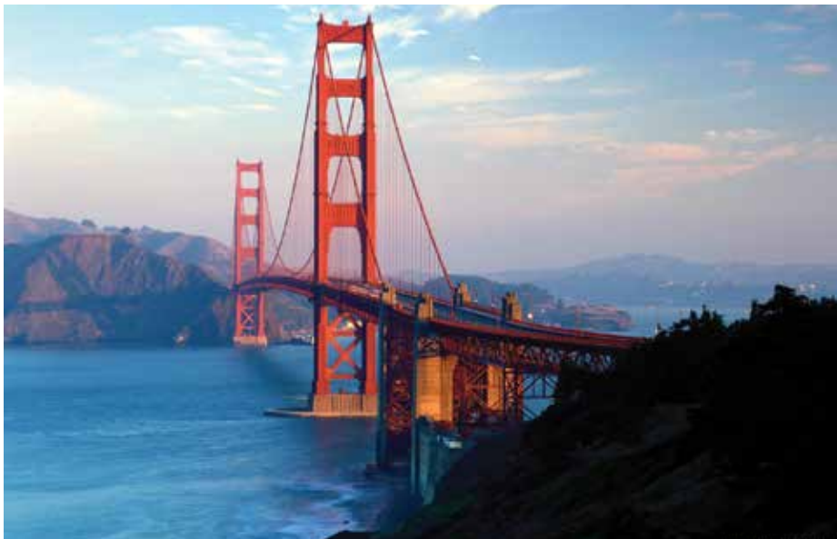
San Francisco's historic Golden Gate Bridge.
