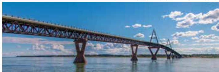
Deh Cho Bridge.
