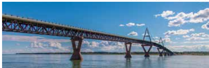
Deh Cho Bridge.
